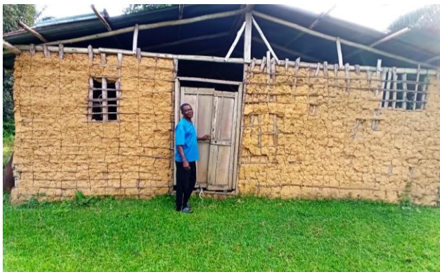
Rev. Tiawroh at J. S. Nagbe UMC in Betu. The church has 1,600 concrete blocks for a new building. Nov. 19, 2023
