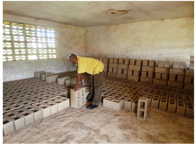
Zwedru UMS principal, Rev. Sam Kanwea, with cement blocks for school's fence. Dec. 1, 2023
