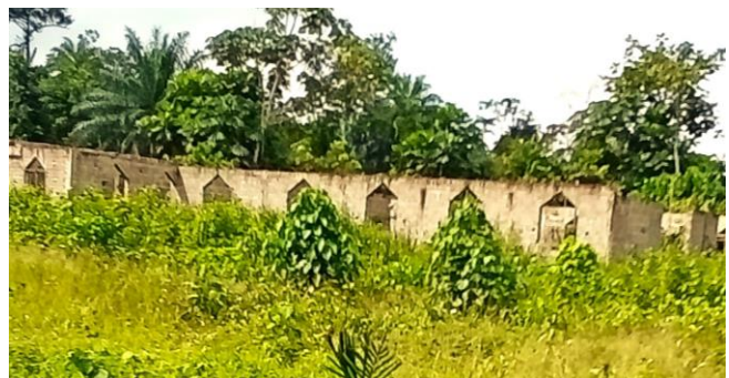
New Toe Gbardee UMC under construction. Dec. 10, 2023.
