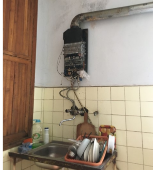
The gas water heater producing tongues of flames
