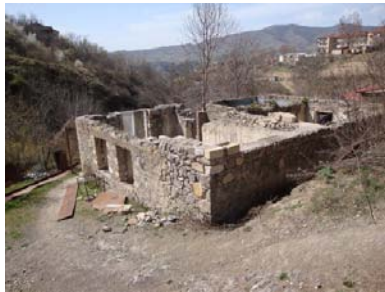
Yura's house after the collapse of the temporary erected roof
