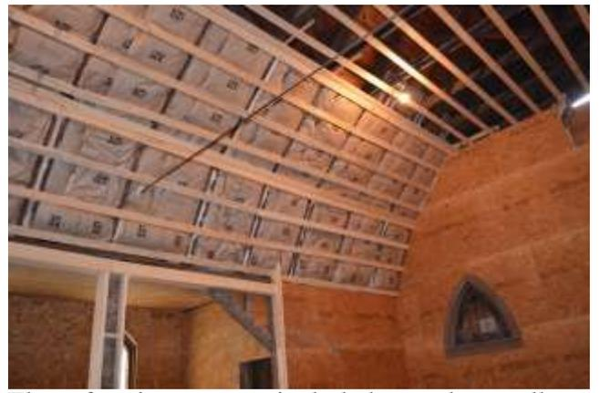
The reframing process included complete wall coverage in OSB plywood. New tie-rods can be seen in the ceiling.
