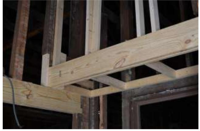
Replaced structural wood framing in the Narthex
