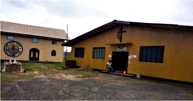
Henri Wilmot Dennis United Methodist School in Topoe Village, Lower New Georgia, was one of the United Methodist Schools that I visited as a WASSCE monitor. Students from Henri Dennis UMS and two other schools took the WASSCE on this campus. The school building is on the right and Lott G. Matthew United Methodist Church is on the left.
