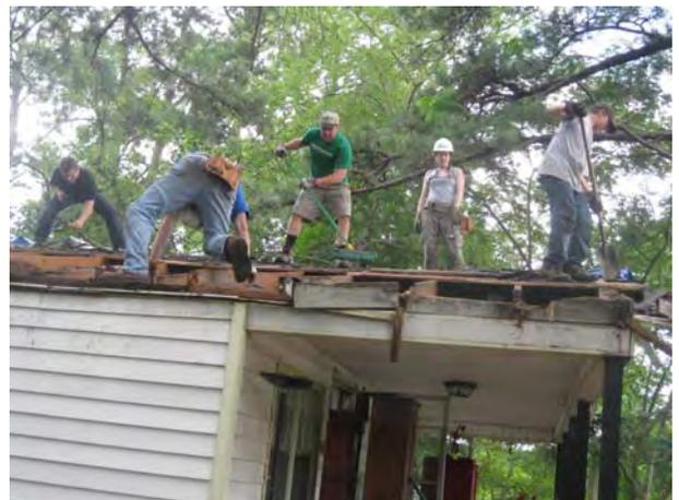
Serious water damage has destroyed the entire roof including the ceiling and floor in the house. Everything, even the rafters and joist had to be replaced in order to begin replacing the roof starting with the sheathing.
