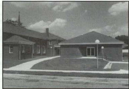
New Fellowship Hall And Educational Building
