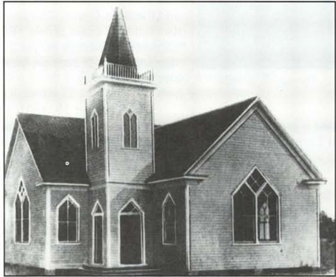
Methodist Episcopal Church South Zebulon, North Carolina
