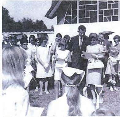
Groundbreaking for the Bell Tower, 1969
