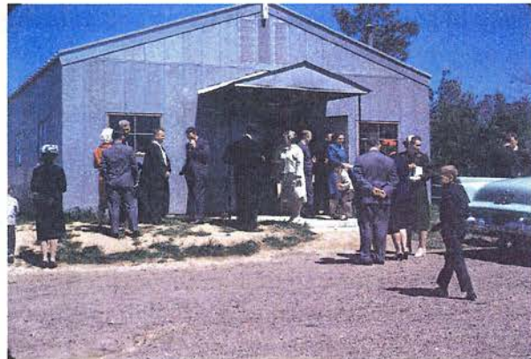
Our First Church, The Metal Building, 1960
