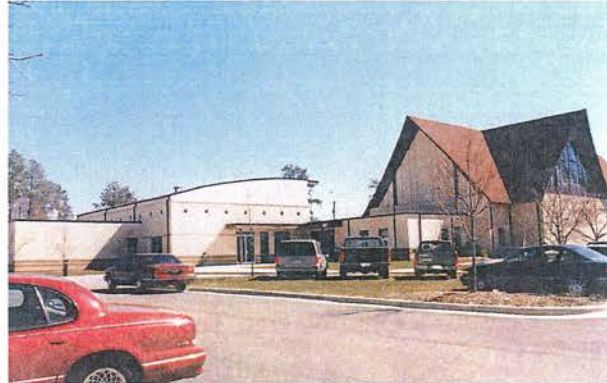
Carson Hall Completed
