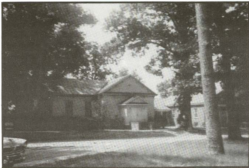
Exterior of the Old Church
