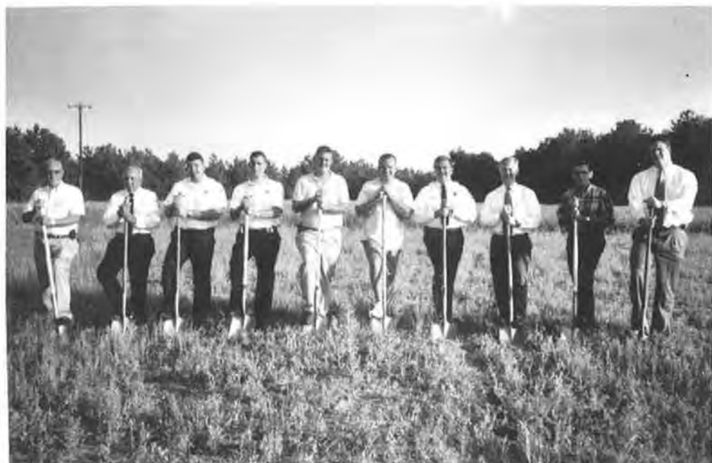
Ground breaking for the Coopers Volunteer Fire and Rescue Department's new station will be on Volunteer Road was May 2003.
