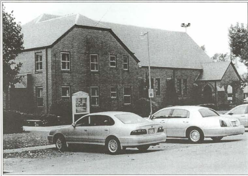
Sunday School Building and Church
