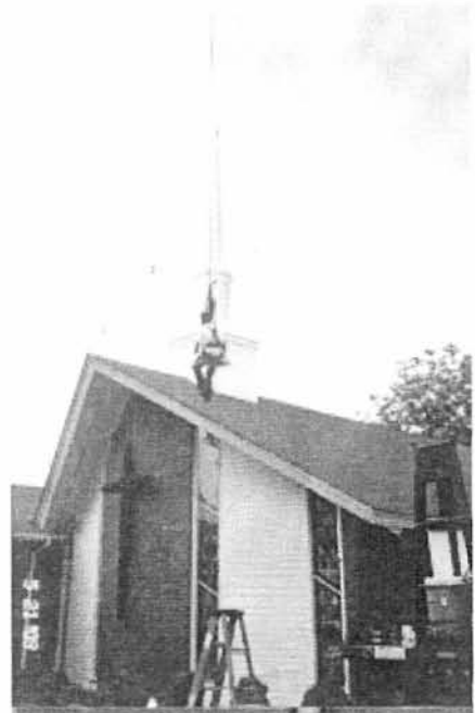
Installer guides new steeple into place in May, 2003
