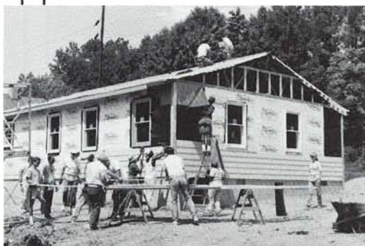
Habitat for Humanity Volunteers constructing Lundsford's new home
