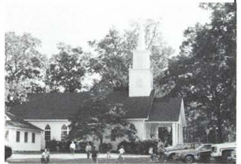
Church Porch and Steeple addition
