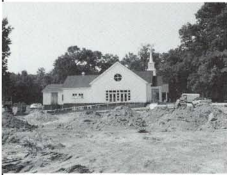
Construction of New Educational Wing - 1988-1989
