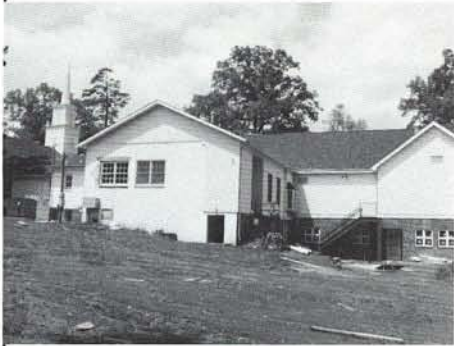
Construction of New Educational Wing - 1988-1989
