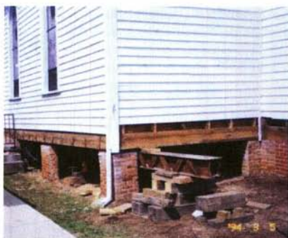
The sanctuary was raised in 1994 to repair the foundation.
