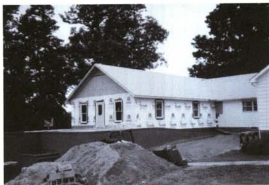
New addition being built in 1998
