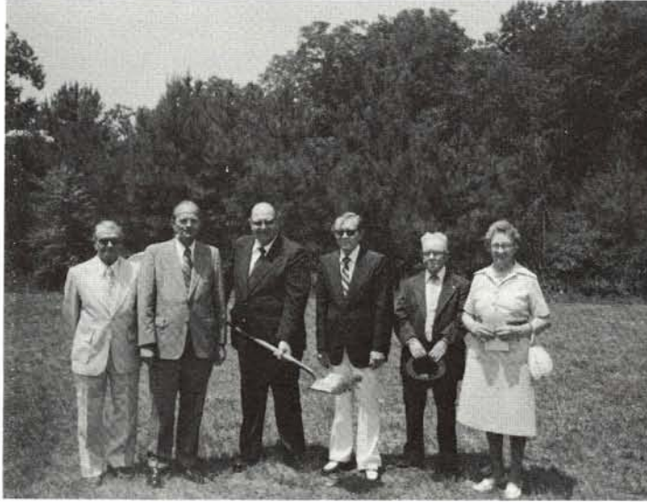
Groundbreaking for our Fellowship Building with Rev. Hardt holding the shovel, with him the District Supt. and Trustees, left to right: Bill Smith, Rev. J. Paul Edwards, Rev. Hardt, Robert Dickinson, Lennie Creech and Ethel Grady.
