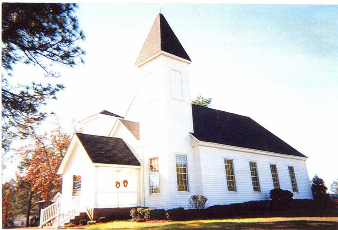
North-side view of Green Lake United Methodist Church After porch was added in September 2003
