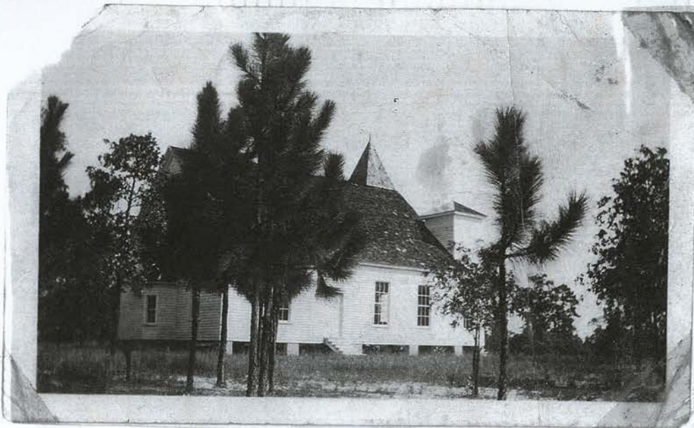
View of the South side (and rear) of Green Lake Church before the Fellowship Hall was built. The following poem is hand-written on the back of this picture. (author unknown)
