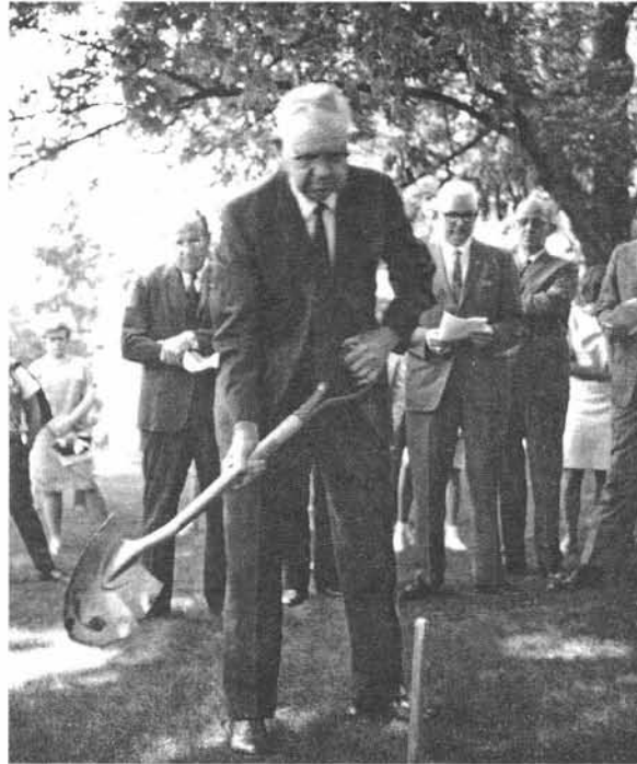
July 17, 1966, Mr. I. I. Henderson at Second Groundbreaking
