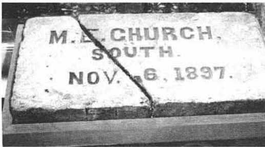
First cornerstone (may have been broken when church burned)
