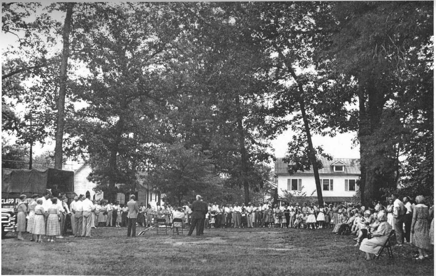
First Ground Breaking, August 7, 1955 (Note left background – old Christian Church, right background – home of a Dr. Moore)
