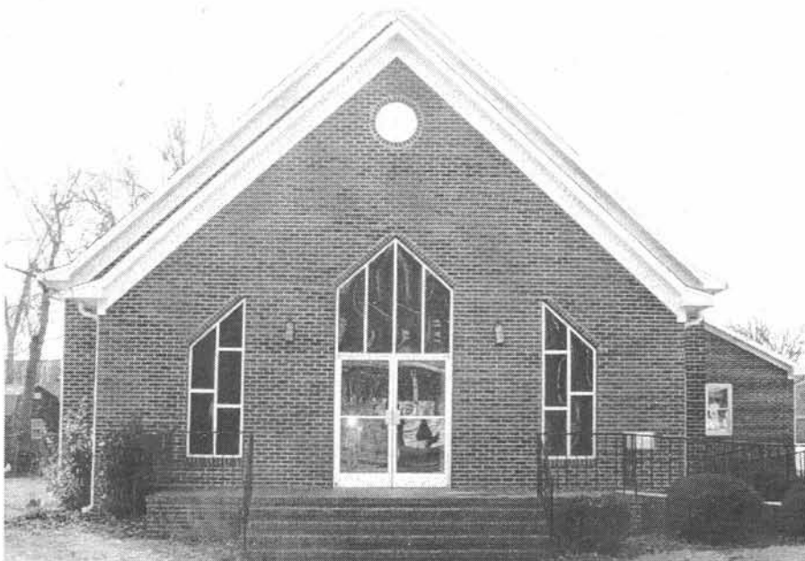
Wayman Chapel A.M.E. Church on North Main Street
