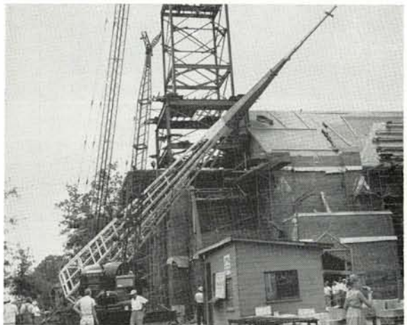
Hoisting the steeple aloft.
