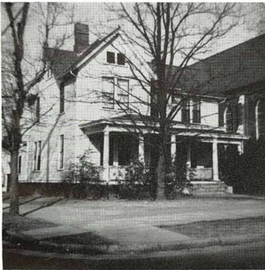
The Old Parsonage. A frame dwelling, believed to have been built about 1895. It stood just west of the old sanctuary, on the corner of Dawson and Edenton Streets, the site where the present sanctuary now stands. It was demolished in 1954, after the New Parsonage was built.
