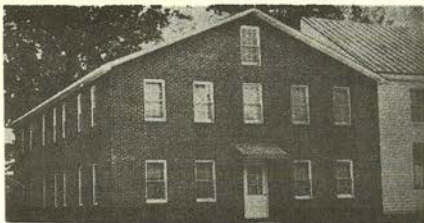
Bundy Hut & Old Education Building
