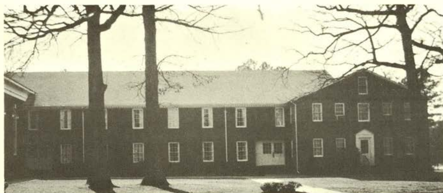
Church School Building
