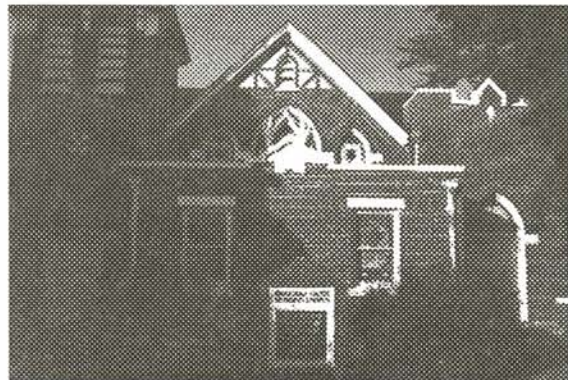
The sanctuary building - 1991
