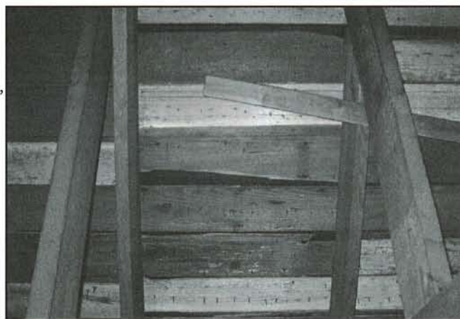
MEMBERS OF BETHANY had always heard that the 1905 church was built using wood from the Old Church. This photograph taken in the sanc- tuary attic of a wide assortment of different boards validates that belief.
