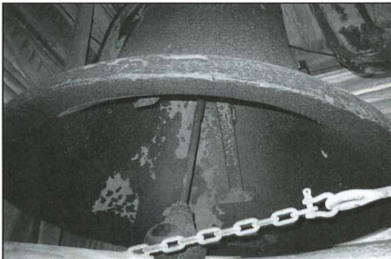
A PICTURE FROM A LOWER ANGLE shows the bell's clapper. Several years ago, the Trustees became concerned that the bell might fall. Mark Nixon shored up the bell and used a chain to strengthen the configuration. (Hughie Basnight photo.)
