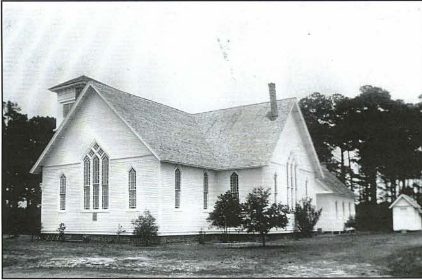
IN THIS RARE PHOTO of Bethany UMC one can see the Skyco church attached to the back of the sanctuary before the two story addition. Note the flatter steeple, the chimneys still in place, the lack of a furnace room, and the block stained glass windows. (Levina Fleming collection.)
