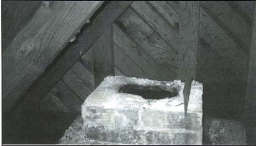
STILL REMAINING IN THE SANCTUARY ATTIC are remnants of the chimneys that were on the east and west ends of the building.
